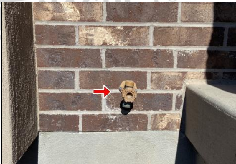
7.3 Item 1(Picture) South side of home
