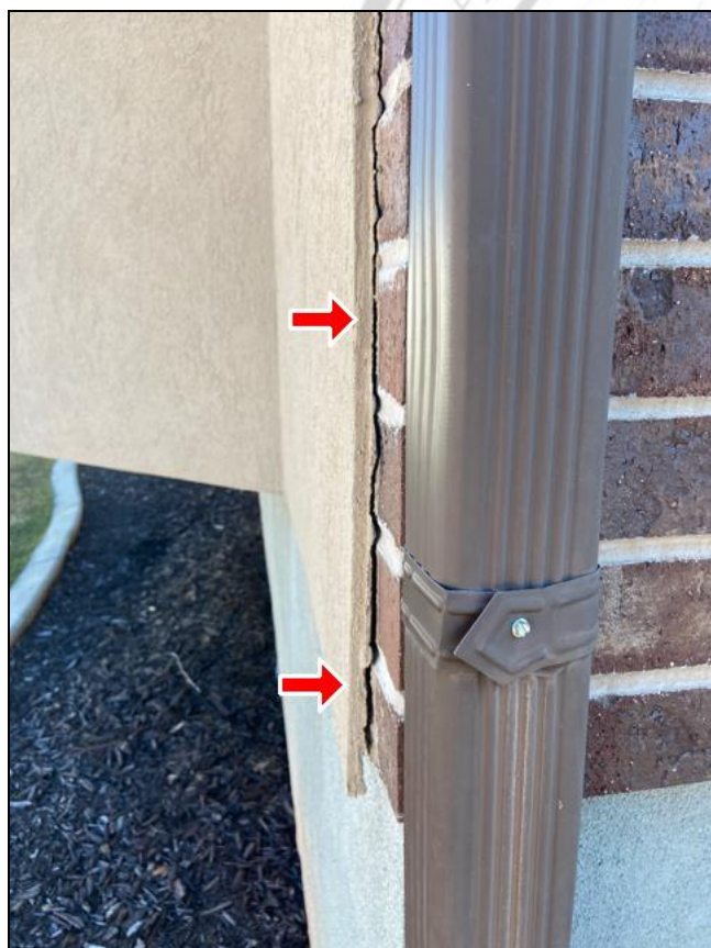
3.2 Item 2(Picture) Northwest corner of exterior
